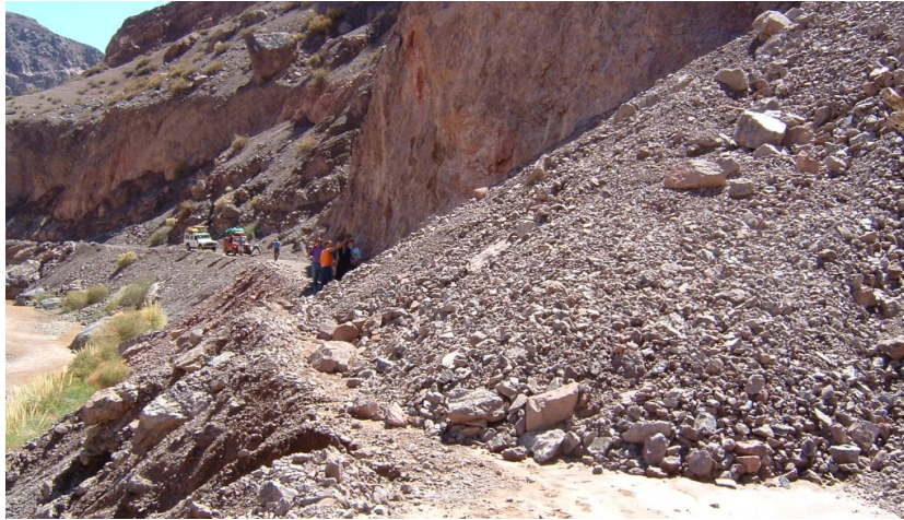
Figure 2.5: Road buried by stones and mud from a landslide after a heavy thunderstorm the day before.
