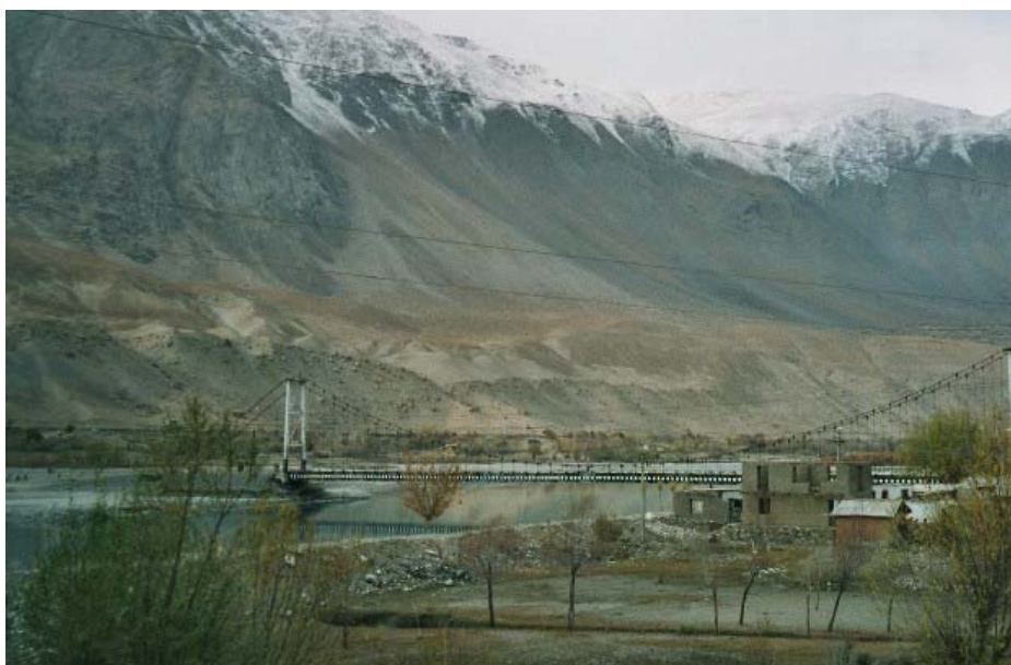
Picture 29: Bridge across the Pyanj river between GBAO and Afghanistan at Roshan (financed by the Aga Khan Foundation)
