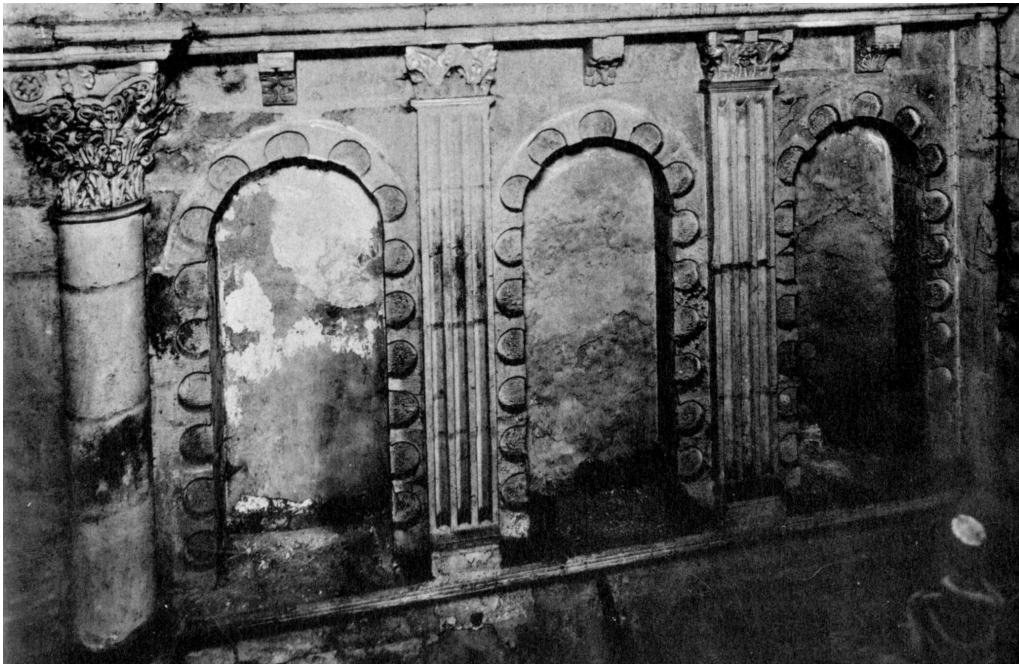
Abb. 3: Nordquerhaus, Westwand, Cluny III.
